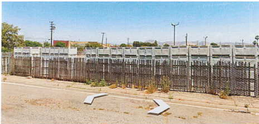
The subject site looking south from Ninth Street.
